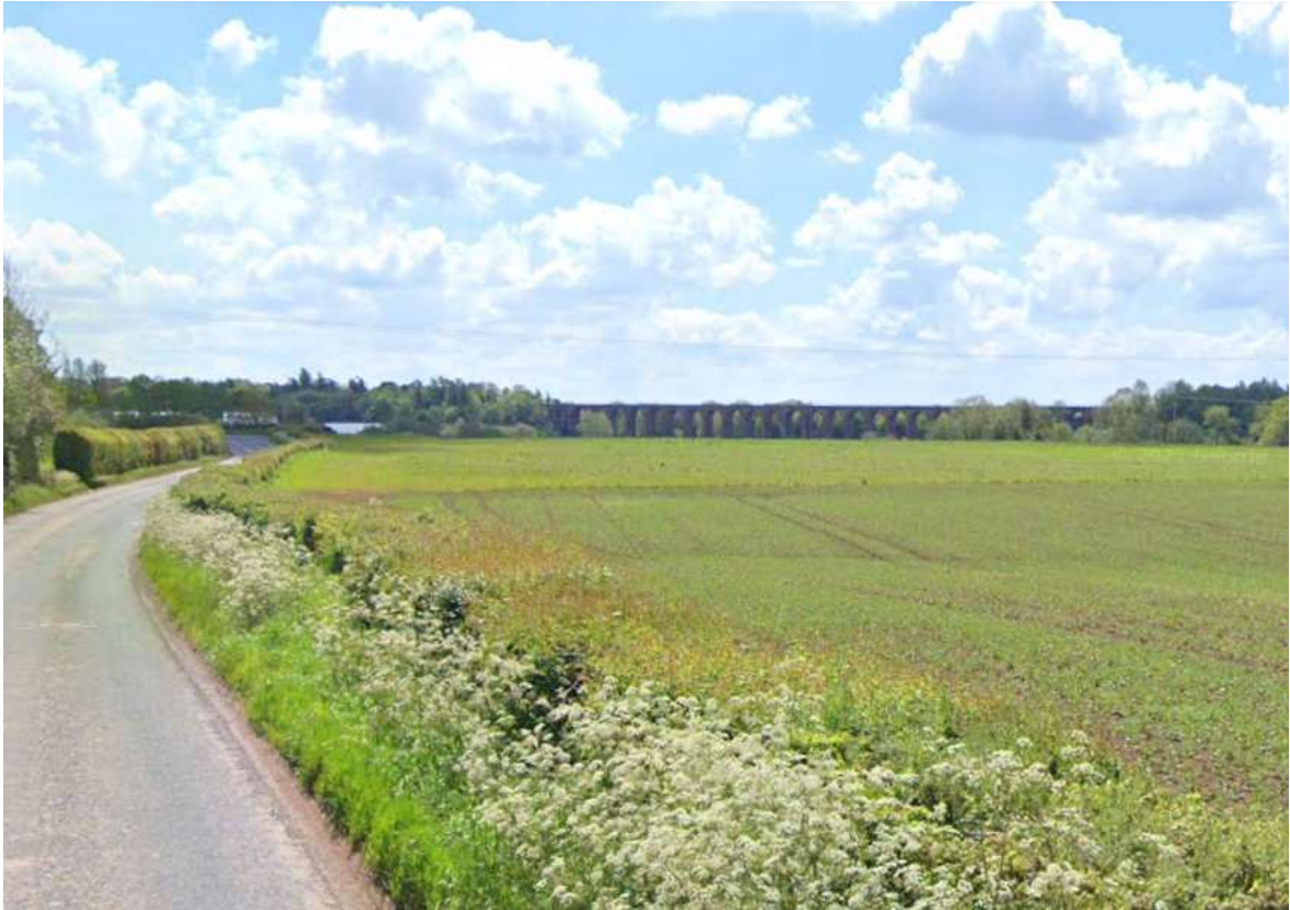
KVR7, looking south east (image © Google)
