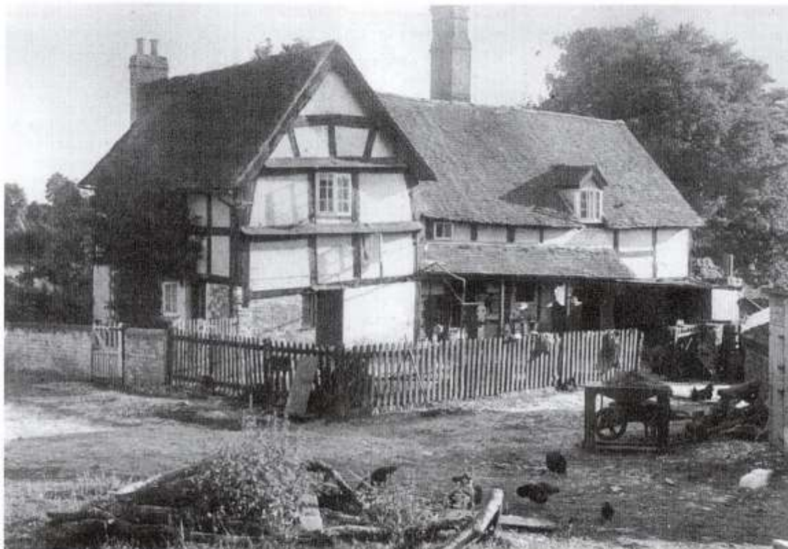
Woodhouse Farm, probably the oldest domestic building in the parish, built not long after the ravages of the Black Death. (HCL/WMC/5173)
